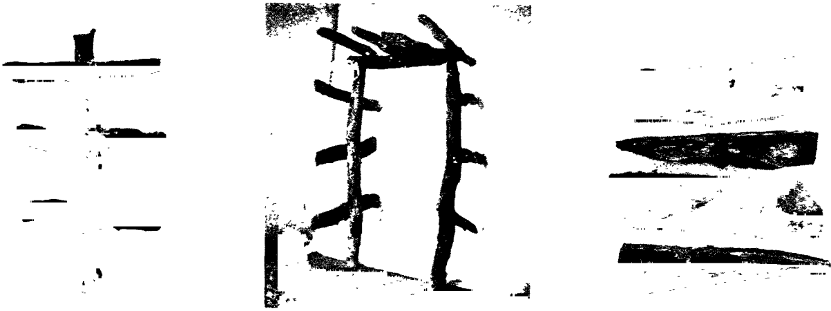
Figs. 340—341. Set of ancient timber consisting of two upright (posts), cross piece (cap), and planks (lagging) above cap and outside of posts.
